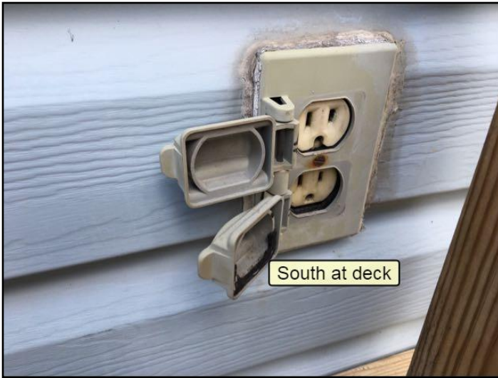
44. No GFCI/GFI (Ground Fault Circuitit...
