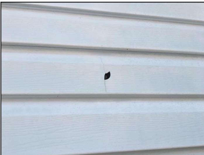
11. Mechanical damage
