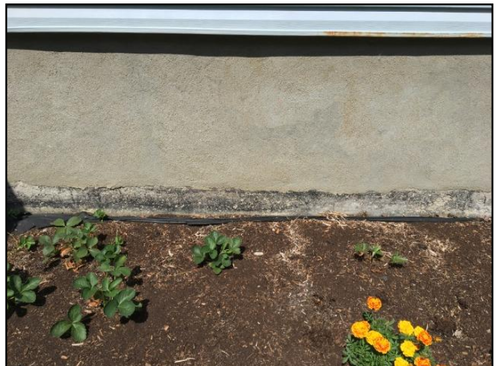
15. Parging damaged or missing
