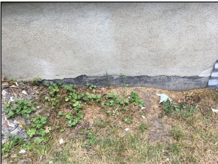
14. Parging damaged or missing
