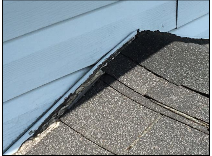
4. Damage, loose, open seams, patched
