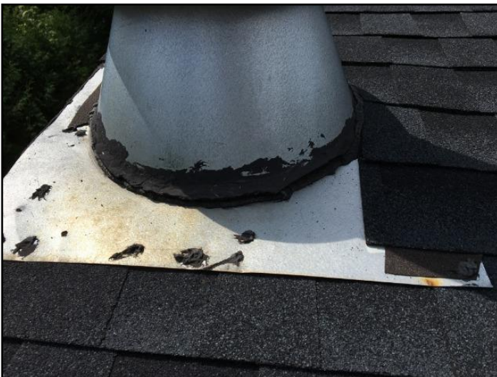
1. Damage, loose, open seams, patched
