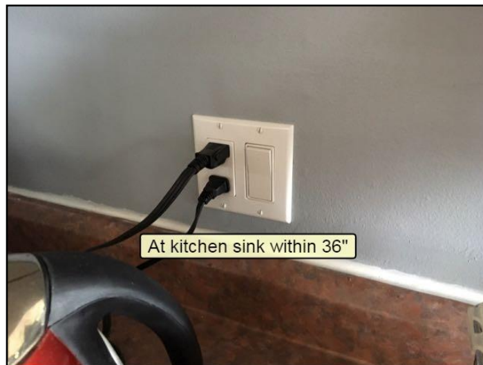
43. No GFCI/GFI (Ground Fault Circuit...
