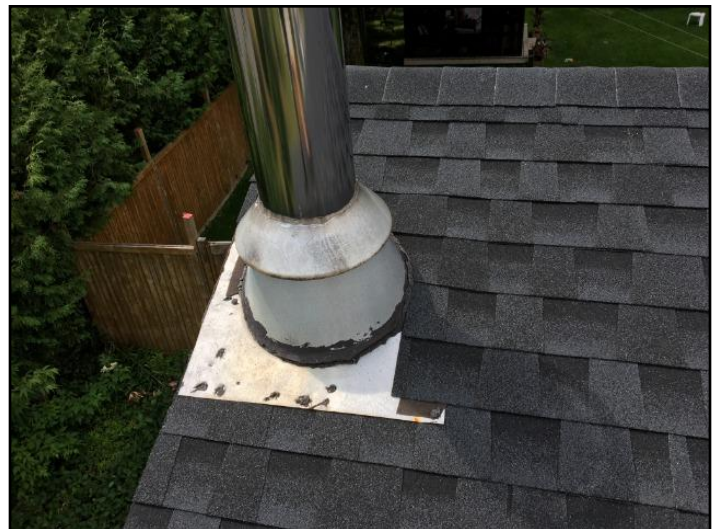
2. Damage, loose, open seams, patched
